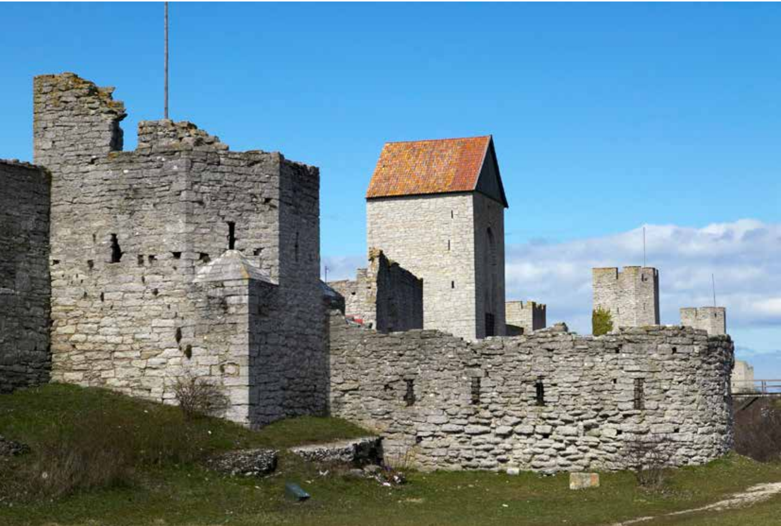
Visby curtain wall with caponier, an extended part of the defences, known as the 'piggy bank'. Photo: Bengt A Lundberg/Raä.
