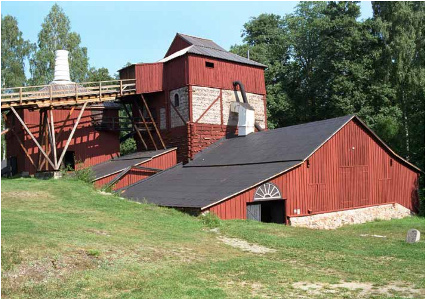
The smelting works at Engelsberg consists of a roasting kiln and a blast furnace. Photo: © Jan Norrman/Raä.
