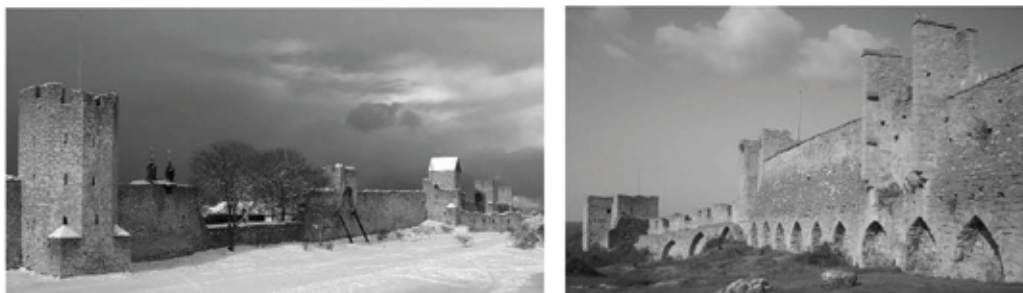
Figure 1: Visby City Wall seen from the outside and the inside. The smaller wall towers ride on top of the wall. Old collapses as well as different kinds of reinforcing structures can be seen in many places.
