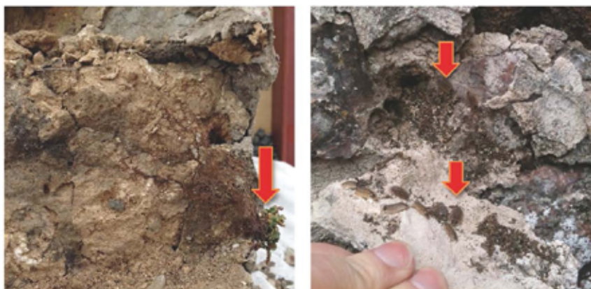
Figure 7. a) A small plant with a large root system reaching far inside the city wall. It has been able to grow first after the joints were repointed with cement mortar. b) Woodlice found in the moist environment behind cement mortar.
