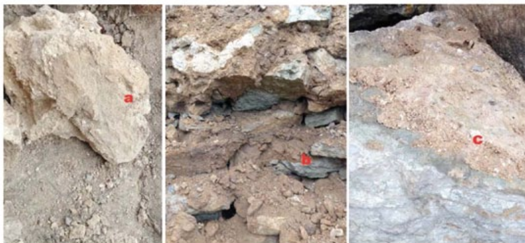
Figure 4. The fat lime mortar (a) is white and rather homogeneous. Lots of smaller lime lumps exist. It has a good adhesion to the limestone. The clay mortar (b) of the wall core is in good condition, powdering when dry and stabile when wet. It has filled up the stone core very well. The type of mortar used in the second building phase (c) has a very good adhesion to the lime stone and is in general extremely well preserved despite its exposed position.
