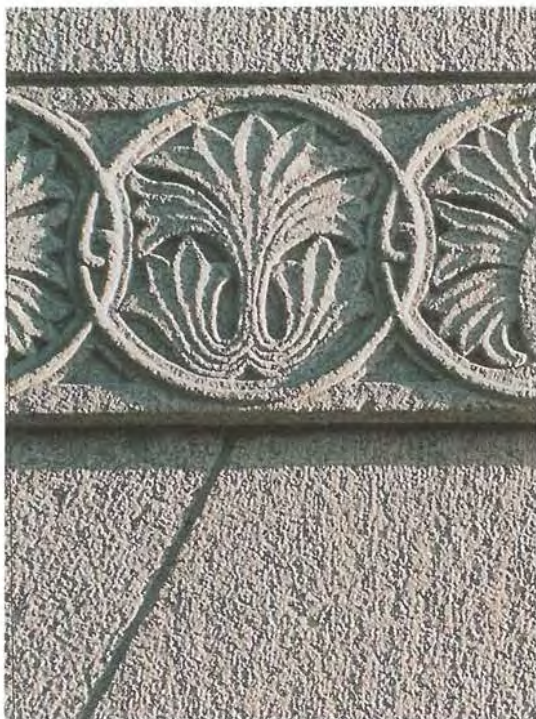
Figur 54. Narvavägen 8, Stockholm, detalj av gradhuggen (krysshamrad) granit med ornament, 1904–09. Foto Bengt A. Lundberg. Narvavägen 8, Stockholm, detail of granite tooled with a bouchard hammer and with carved ornaments, 1904–09.
