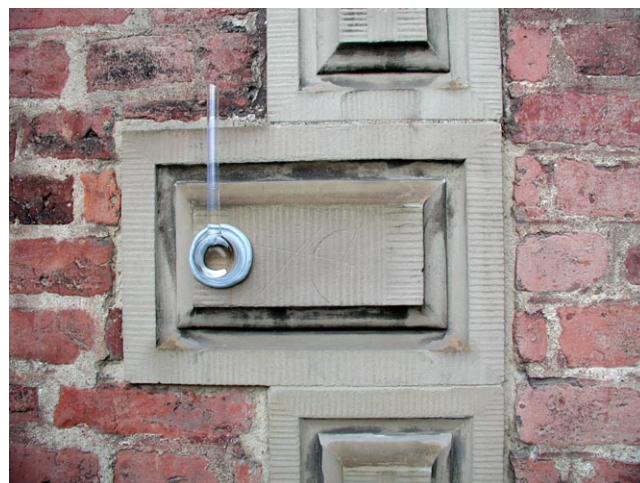
Figure 2. Measurement with Karsten pipe at Riddarhuset.
