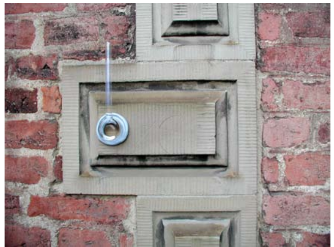
Figure 2. Measurement with Karsten pipe at Riddarhuset.
