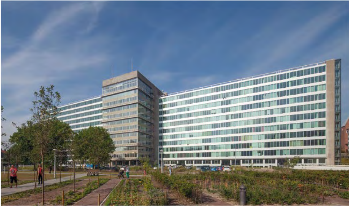
THE 1960 GAK BUILDING after conversion into housing, featuring a re-designed aluminium-and-glass curtain wall that looks almost exactly like the original. Photo: Luuk Kramer.
