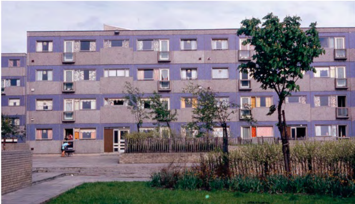
FIGURE 6. GLASGOW, SCOTLAND. Mass housing in the Anderston Cross Comprehensive Development Area: phase 1, built 1965–67 using the Bison precast concrete panel system. Planned as part of a 1960s' regeneration of the area to replace traditional stone-built tenements, this development has itself been largely remodelled and rebuilt as part of an ongoing regeneration programme, in which none of the four values of community, resource, usefulness and cultural was taken into account. This photograph was taken in 1970. Photo: Dennis Rodwell.
