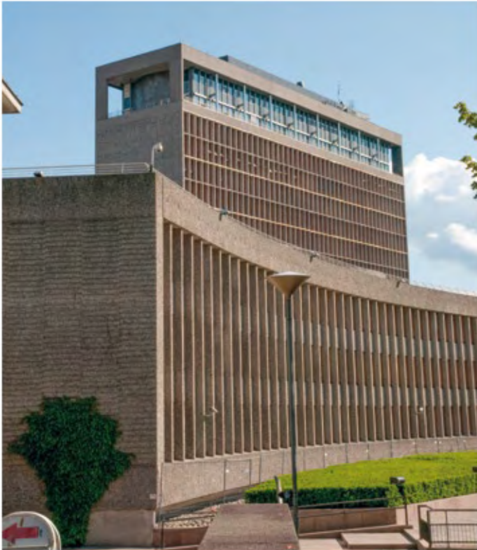
THE H BLOCK AND THE Y BLOCK of the Government Quarter. Photo: Trond Joelson, Byggeindustrien.
