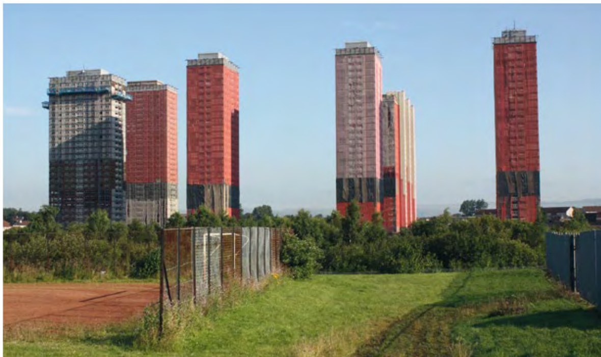
FIGURE 5. GLASGOW, SCOTLAND. Programmes of demolition of 1960s and '70s residential tower blocks in the city began in the early 1990s. At the time of their erection, 1964–69, the eight blocks of the steel frame construction Red Road flats were reputed as the tallest buildings in Europe (two slabs of twenty-eight storeys, four point blocks and two tower blocks of thirty-one storeys; designed 1962; Sam Bunton & Associates, Architects). Designed for a population of 4 700, the lack of communal facilities contributed to a number of problems on the estate. Options for regeneration were not considered. One slab block was demolished in 2012 and one point block in 2013. This photograph shows the remaining six blocks being prepared for demolition in late 2015. Photo: Dennis Rodwell.
