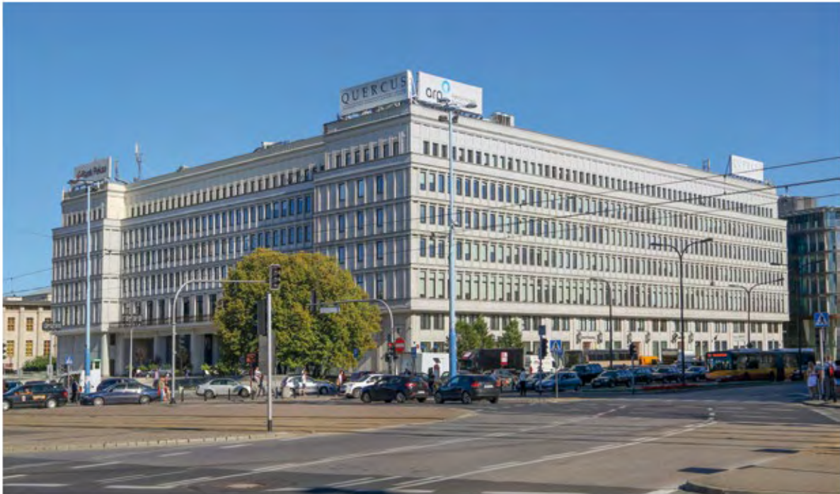
WARSAW. POLISH UNITED WORKERS' PARTY CENTRAL COMMITTEE BUILDING (W. Kłyszewski, J. Mokrzyński, and E. Wierzbicki, 1947–1952). State in 2016. Photo by P. Kobek from the Collection of the National Heritage Board of Poland (hereinafter referred to as Coll. NID).
