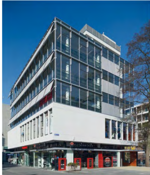
THE 1953 HUF BUILDING after restoration. Sunscreens have been added in order to allow for clear glazing. Photo: Jannes Linders.
