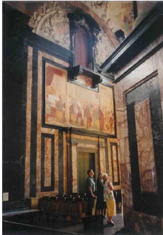
Church of St. Virgin Mary's Visit in Kamalduliai Convent of Pazaislis. Electrical under-floor heating.
