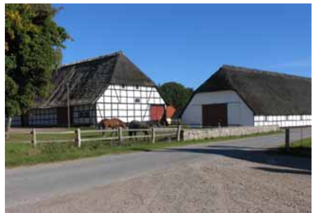
Figure 5. The manor has received financial help from the Danish national heritage preservation authority in order to finance the repair of its unusually large thatched roofs.
