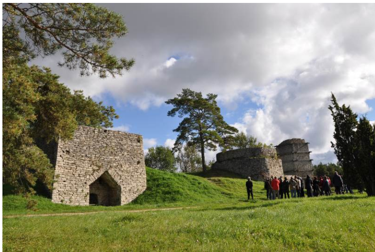
The lime-works of Barläst. Photo: Helen Simonsson
