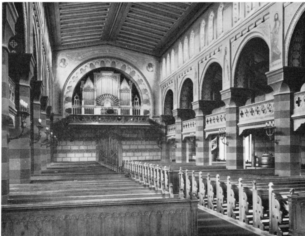
Fig. 13. Interiör mot v. Inneres gegen Westen. Interior towards the west.
