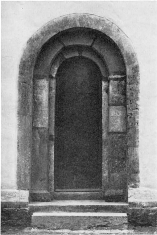
Fig. 110. Tornets N portal. Foto 1963. S. 101. N Portal des Turms. N door of tower.
