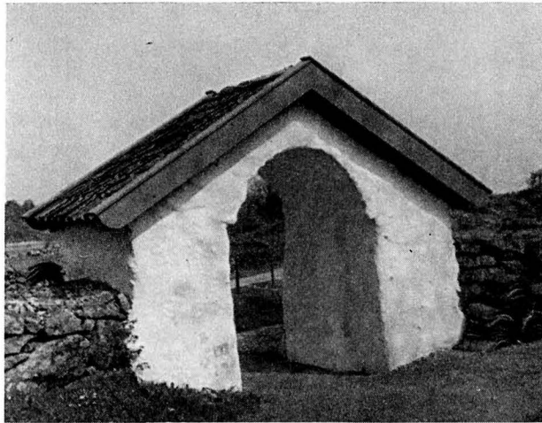
Fig. 317. Stiglucka i kyrkogårdens N mur. Foto U. Larsson 1956. N Kirchhofportal. Lich-gate in N wall of churchyard.
