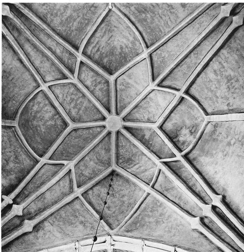
Fig 23. Senmedeltida valv i koret, s k sturevalv. Foto 1969. Late medieval vault in chancel, so-called Sture vault.
