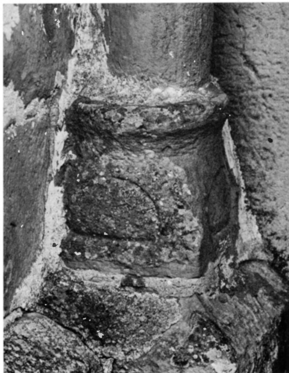
E colonnette base of N portal of nave.
