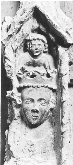
Fig 59–65. Stora kapellets portal.
