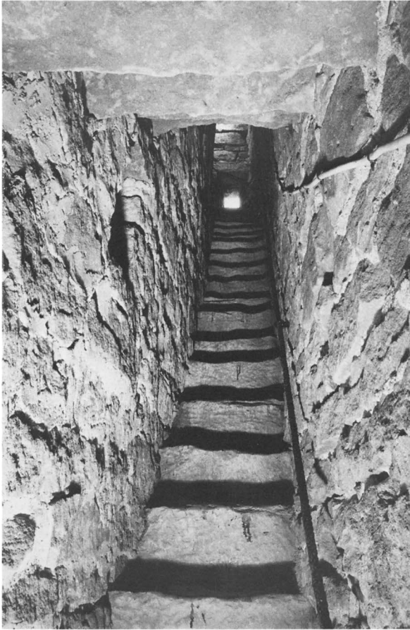
Fig 30. Ursprunglig trappa i tornets norra mur. Foto 1977. Original staircase in the north wall of the tower.
